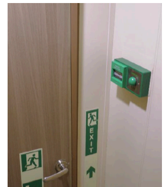
Exit buttons are used to de-activate magnetic locks
